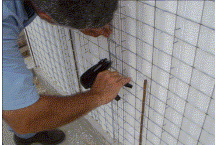
Photo 3: Manual clamping tool for connection of wire mesh.
